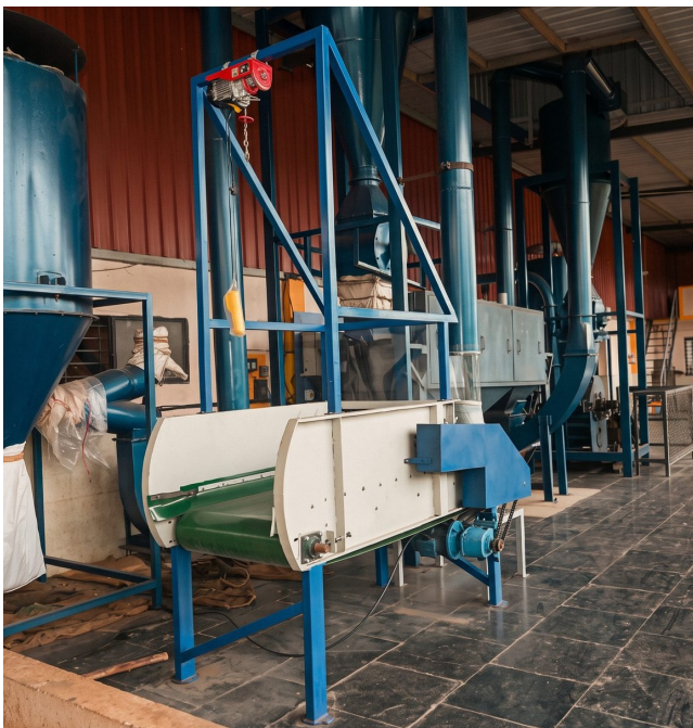
Grinding and milling hall
